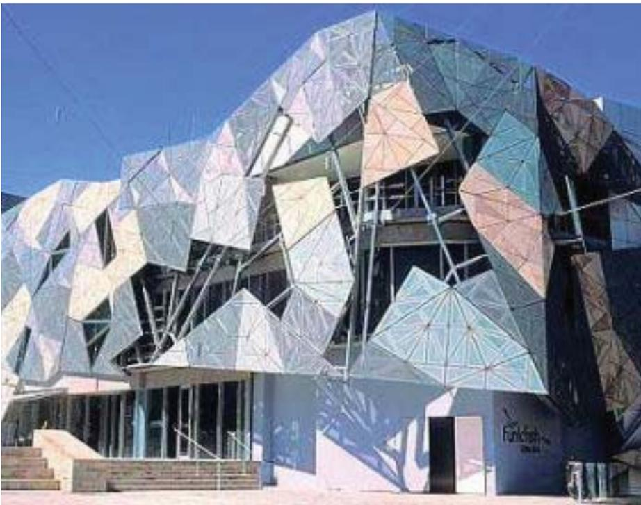
figures 11 and 12: lab architecture's Federation Square in Melbourne. Small triangles form bigger triangles forming facade systems
