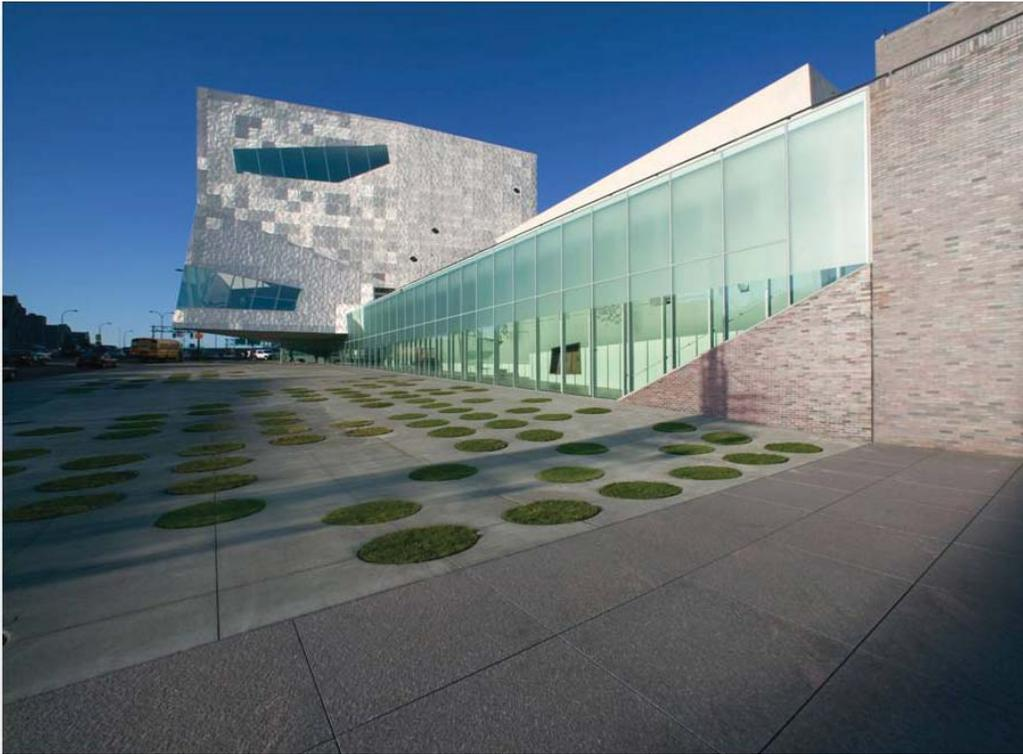
The Walker Art Center addition, with its floating volume clad in crumpled aluminum panels
